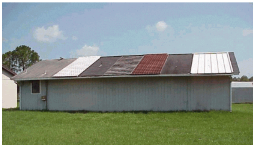
Figure 4. Flexible Roofing Facility during 2001 summer testing; South exposure.
