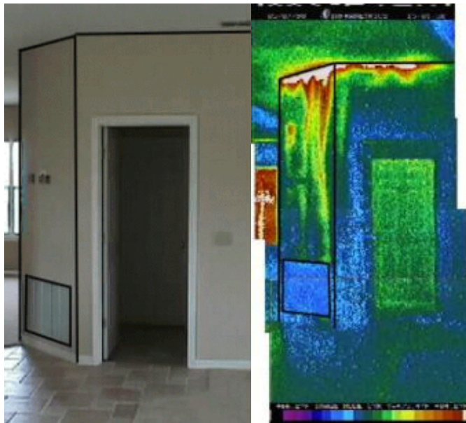
Figure 2. Thermograph of air being drawn from the attic to the air handler in a Florida house.
