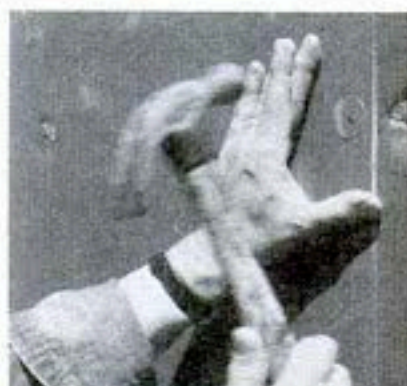
ATTACH BOARD to furring strips or studs with nails and roofing washers
