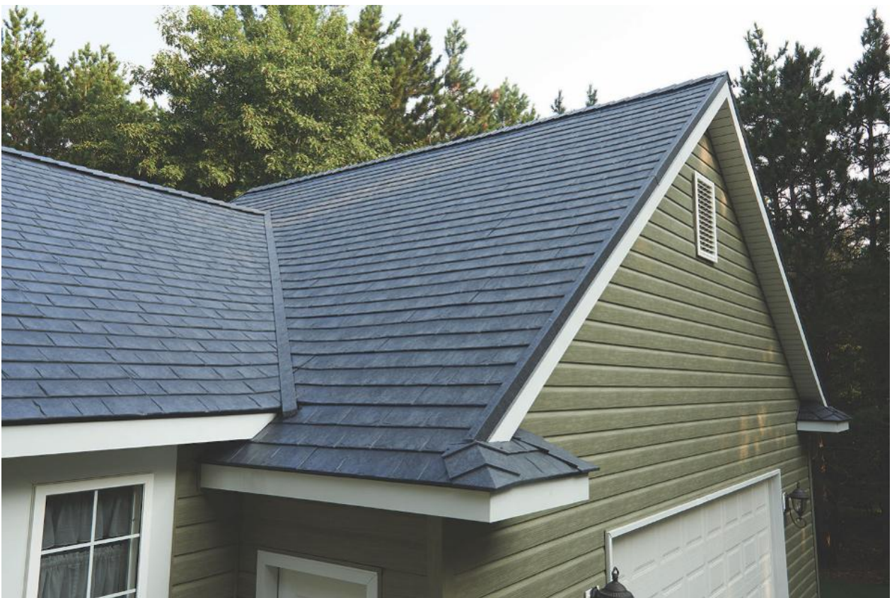
The metal tile roof looks like slate but is metal produced by CertainTeed. PHOTO COURTESY OF CERTAINTEED.
