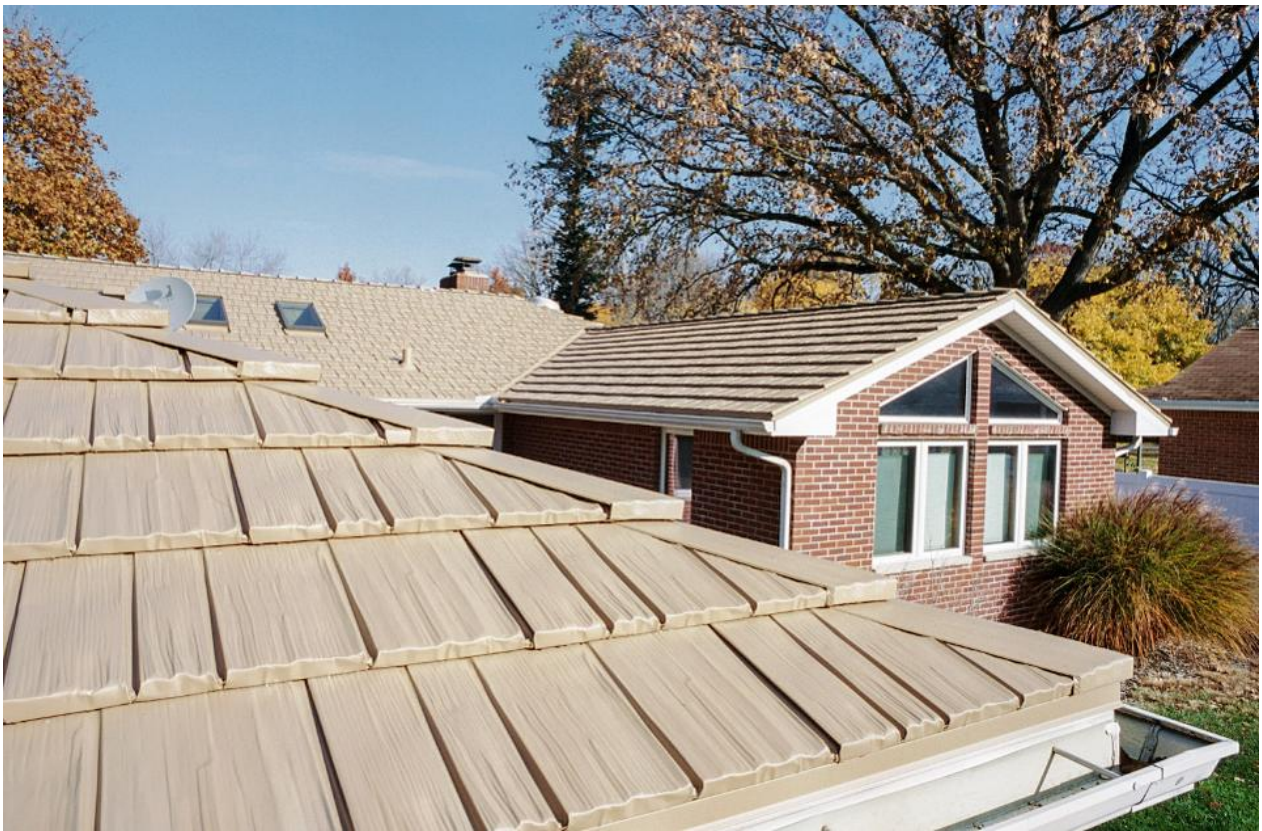
This metal tile roof has the look of a shake roof but will be far more durable and long lasting. PHOTO COURTESY OF ISAIAH INDUSTRIES.
