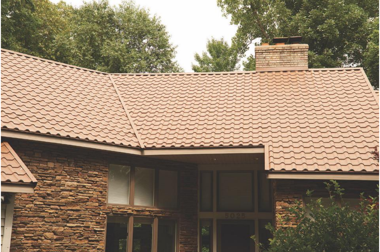
Matterhorn Tile by CertainTeed replicates the classic look of a Tuscan villa, with a steel manufacturing process that makes it both lighter and stronger than standard clay tile. PHOTO COURTESY OF CERTAINTEED
