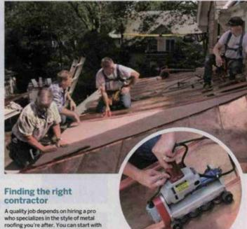
Top: At TOH's Arlington Arts and Crafts project. Tom Silva and Kevin O'Connor get an up-close look at the standing-seam portico roof installation. Each copper panel is laid over a slip sheet and fastened with copper nails; then an electric seamer (inset) crimps panel edges for a tight, no-leak joint.
