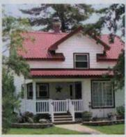
TILE LOOK These 38-inch-long panels have the thick profile of six clay tiles, but not the weight, fragility, or fussy installation of fired clay. A low-gloss PVDF finish and a special embossing technique help approximate the real thing. Shown: Met-Tile Metal in Bravo Red, from \$3 per square foot; mcelroymetal.com
