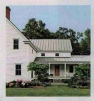
STANDING SEAM Its crisp lines, formed where panel edges interlock, complement a wide variety of houses, from traditional to modern. Hidden clips hold panels in place and let the metal move. Similar to shown: Universal Standing Seam in Silverstone, from \$2.75 per square foot; greenamericanhome.com
